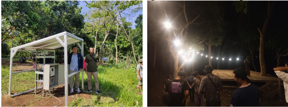
Figure 6. Results of Garden Lighting Installation and Test at Night
