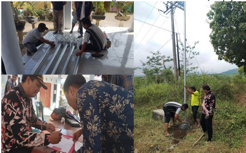
Figure 7. Installation Process and Training on Use and Maintenance of PJU Equipment
