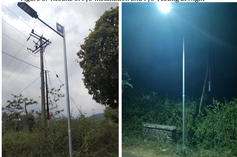
Figure 8. Results of PJU Installation and PJU Testing at Night
