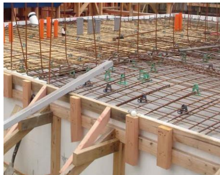
Figure 3.1 Wooden materials for conventional formwork
