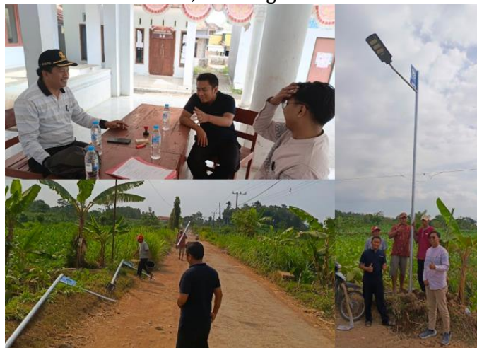
Figure 6. Installation Process, Training on Use and Maintenance of PJU
