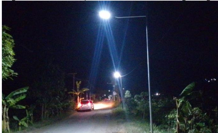
Figure 7. Results of PJU Installation and Testing at Night
