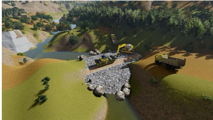
Figure 7. Visualization of Excavation Work
