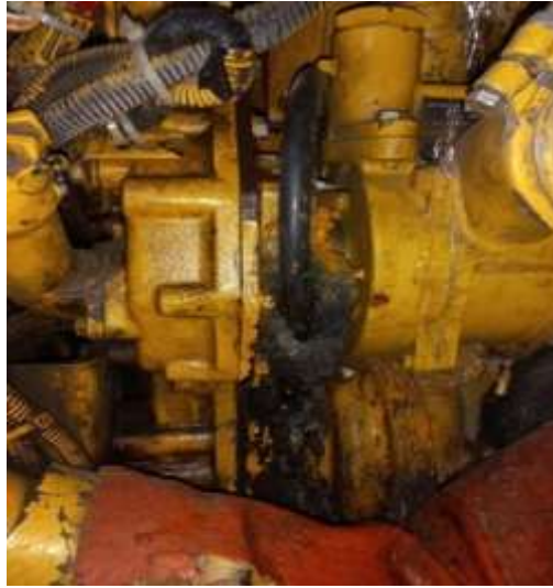
Figure 2 Cracked Sea Water Pump Cover Source: Processed Research Data (2024)
